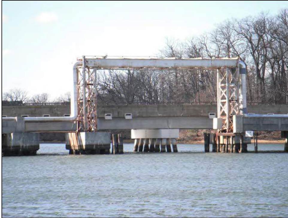
Figure 1-1 Utility Bridge, West View
