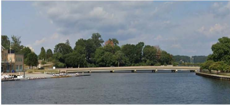
Decatur Avenue Bridge, east view
